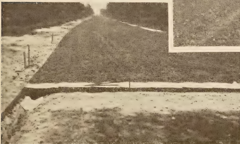
FIGURE 3.—MIXED-IN-PLACE CONSTRUCTION
